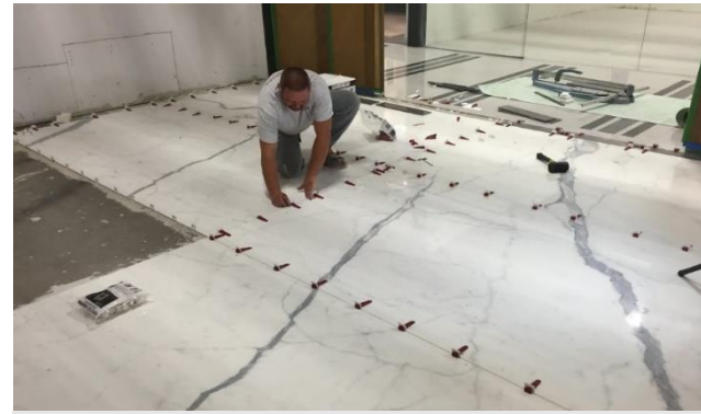
Large, thin, slab tiles can be 6mm thick
