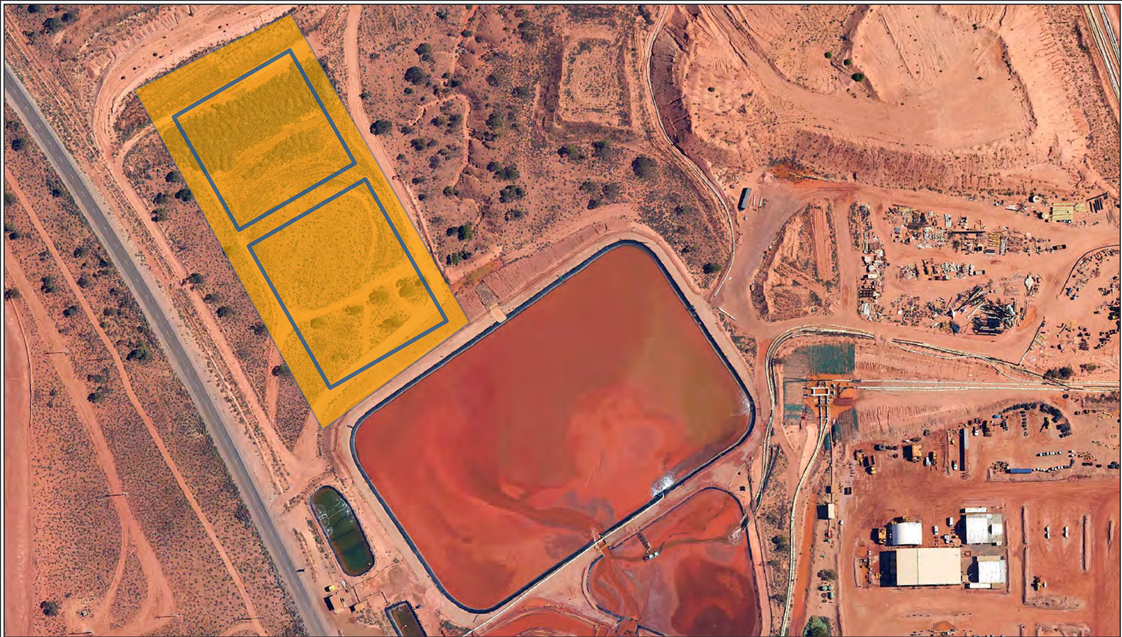
Figure 3-2: Turkey's nest and collector pond location
