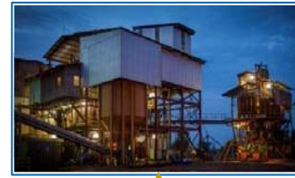
Mineral Separation Plant separates the heavy mineral concentrate – installed capacity to produce in excess of 200,000 tpa
