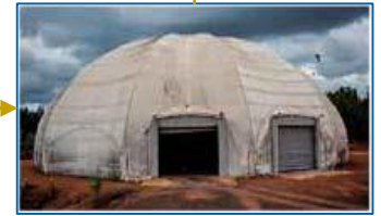
Silos and domes for product storage
