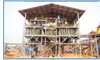
Concentrator plants to process the dry mined ore into a heavy mineral concentrate
