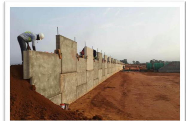
R.O.M Tip Retaining Wall Panels
