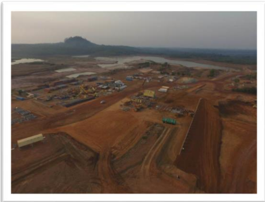
Aerial View of Plant Terrace & Site Establishment Area
