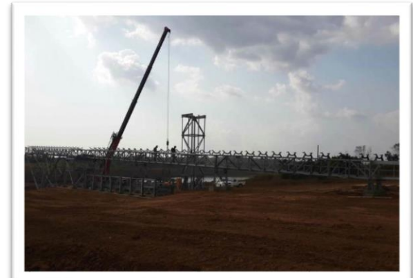
Oversize Conveyor Structure
