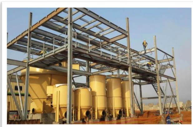
Spiral Building & Sumps
