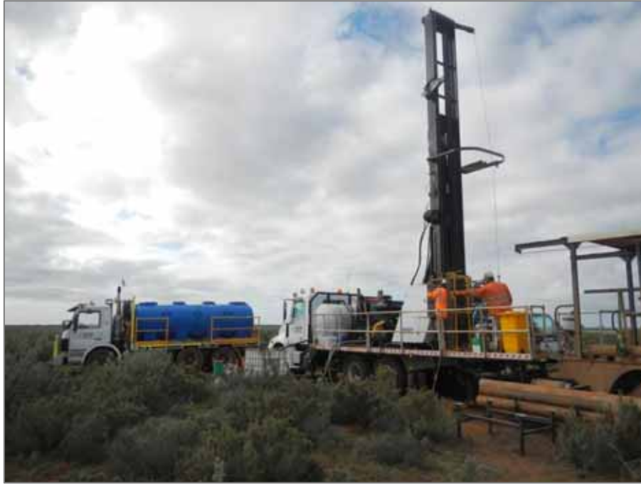
Figure 2: Sonic drill rig at WBGEC-1 bore hole site.
