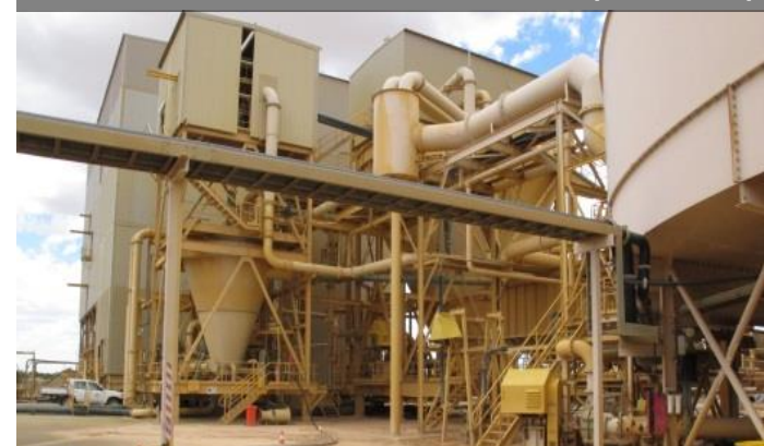
Newman Wet Concentrator Plant (Eneabba)
