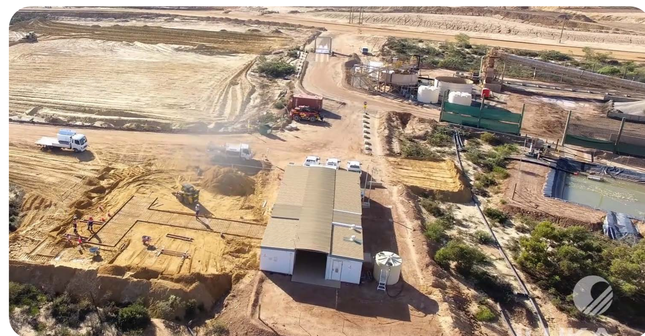
June 2021 construction progress on schedule
