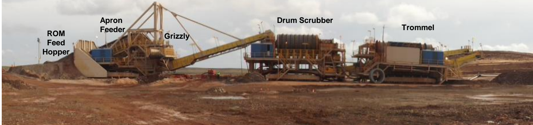
Wet Concentrator Plant
