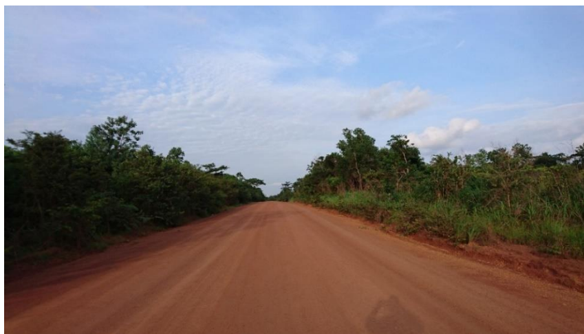
Haul roads in the SR Area 1
