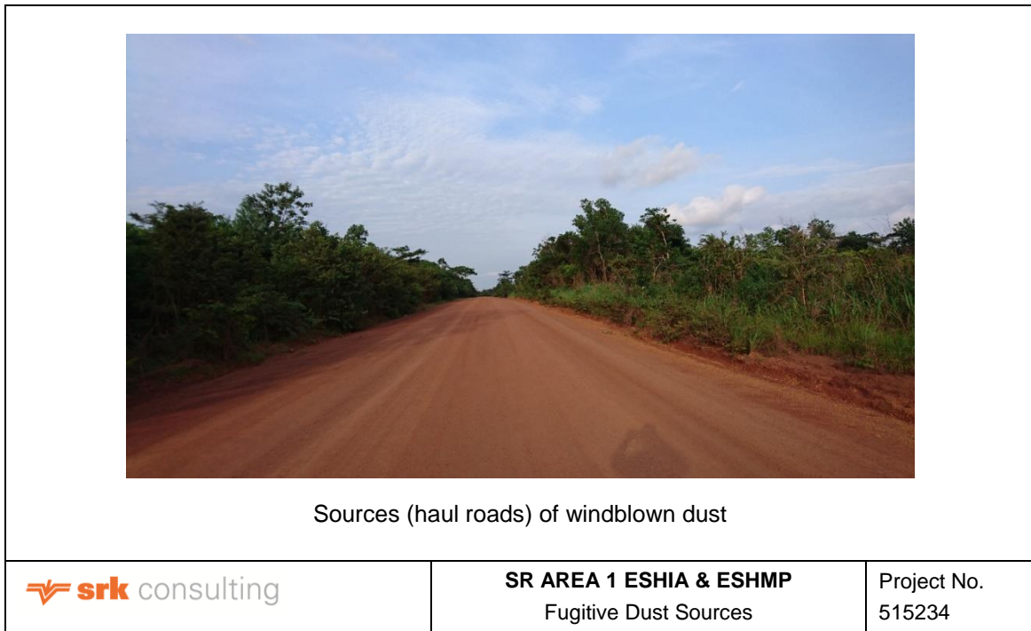
Figure 7-3: Fugitive dust source within the SR Area 1
