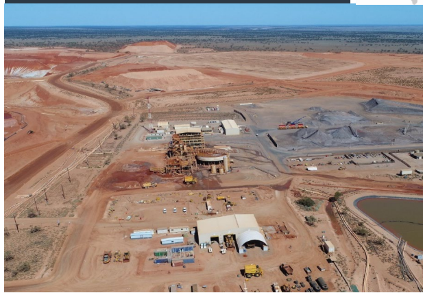
Jacinth-Ambrosia is one of the world's largest zircon mines, discovered and developed by Iluka and operating since 2009. Narngulu mineral separation plant processes Jacinth-Ambrosia and Cataby non-magnetic products.
