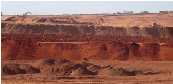
Rehabilitation in Cell 1 West
