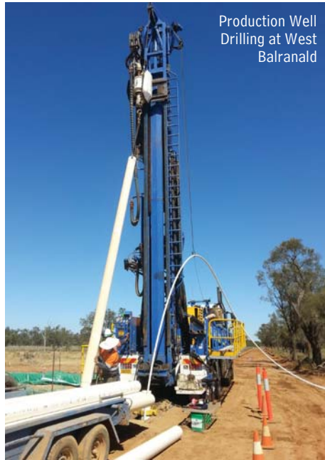
Reinjection bore at long-term pump test site
