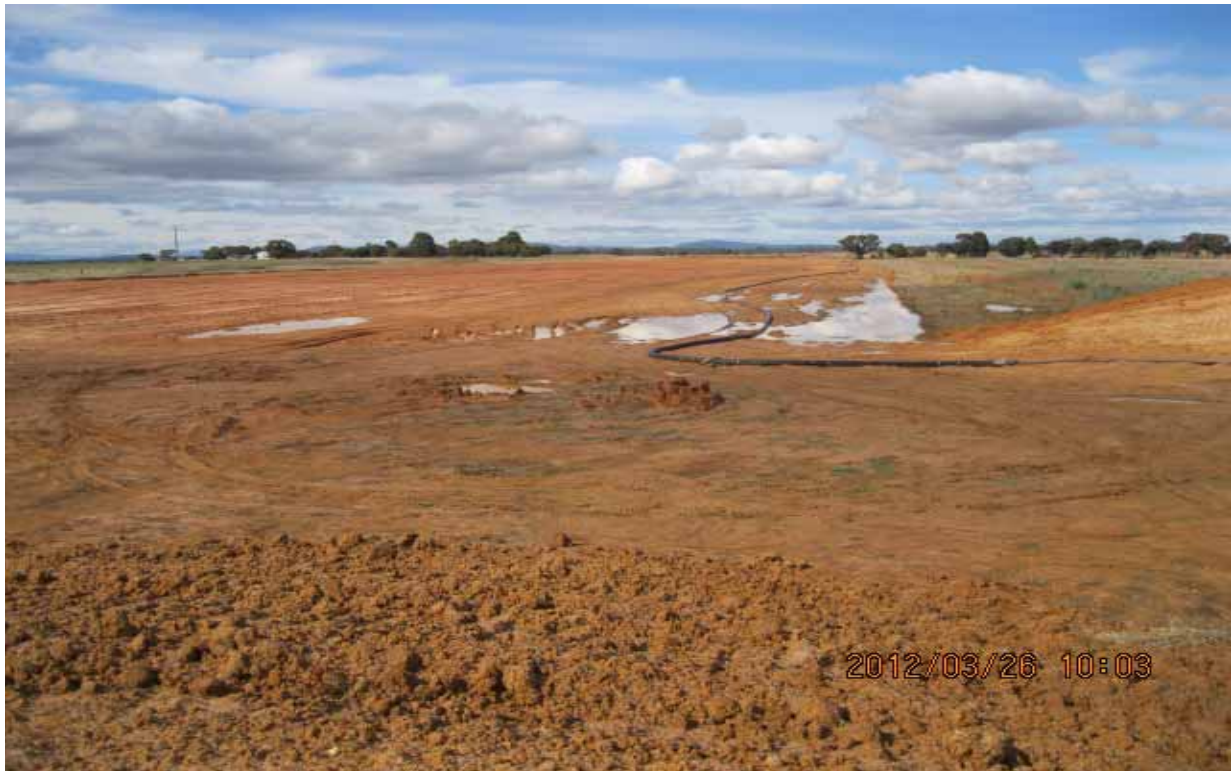
Plate 11: Earthworks at Echo mine showing backfilled area prior to shaping and replacement of subsoil and topsoil
