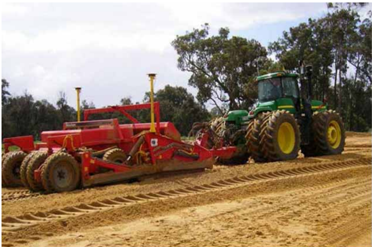
Plate 12: 1 GPS fitted carry-grader and tractor at Jacinth Ambrosia mine
