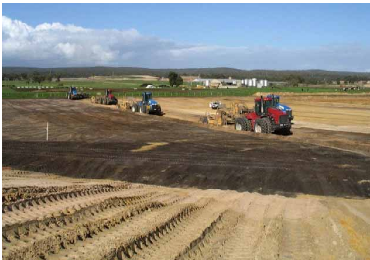
Plate 14: Soil replacement operation at Echo mine
