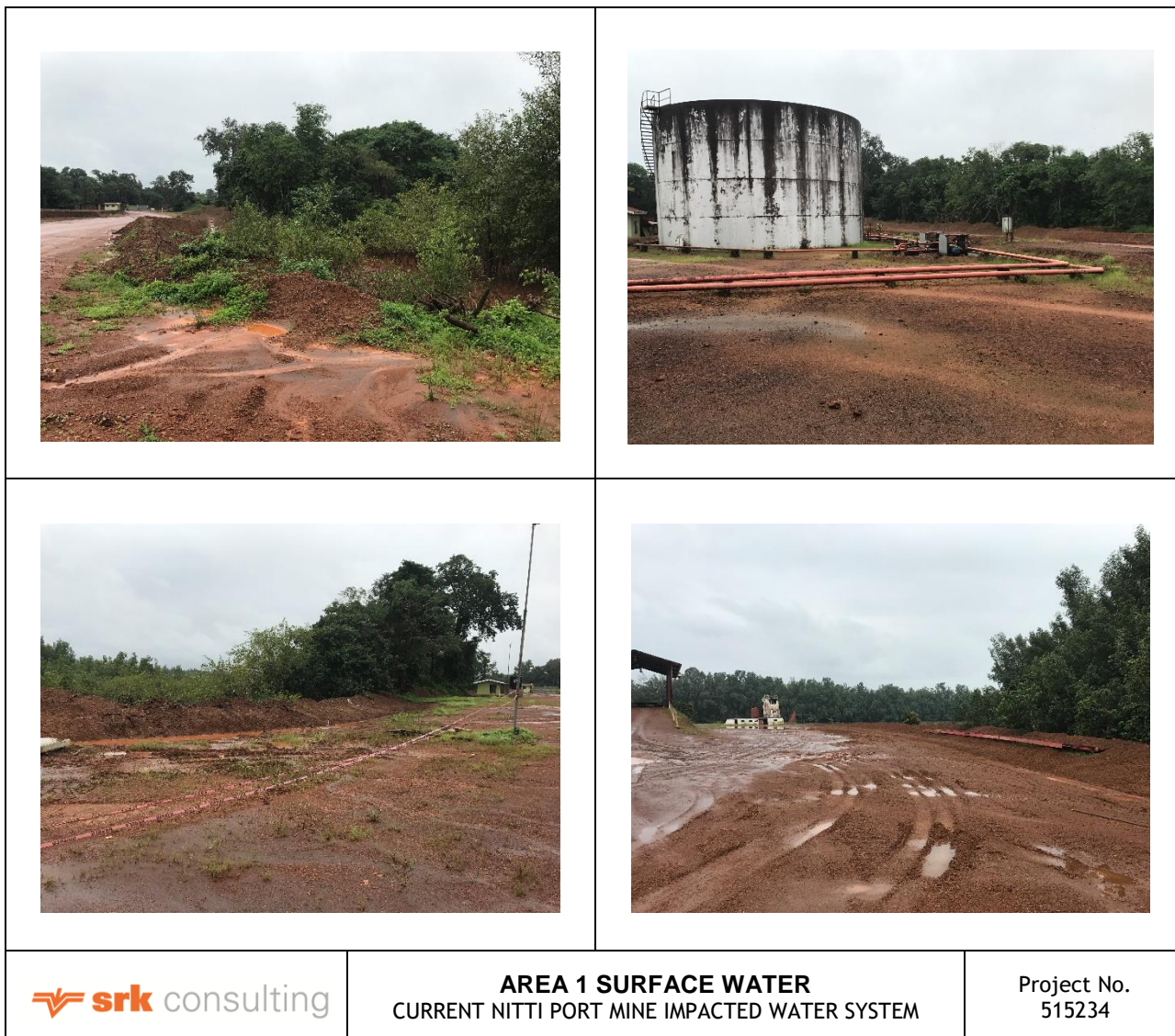
Figure 7-17: Photographs of the current Nitti Port mine impacted water system showing the mine impacted water collection drains and the earthen berms around the fuel storage tanks
