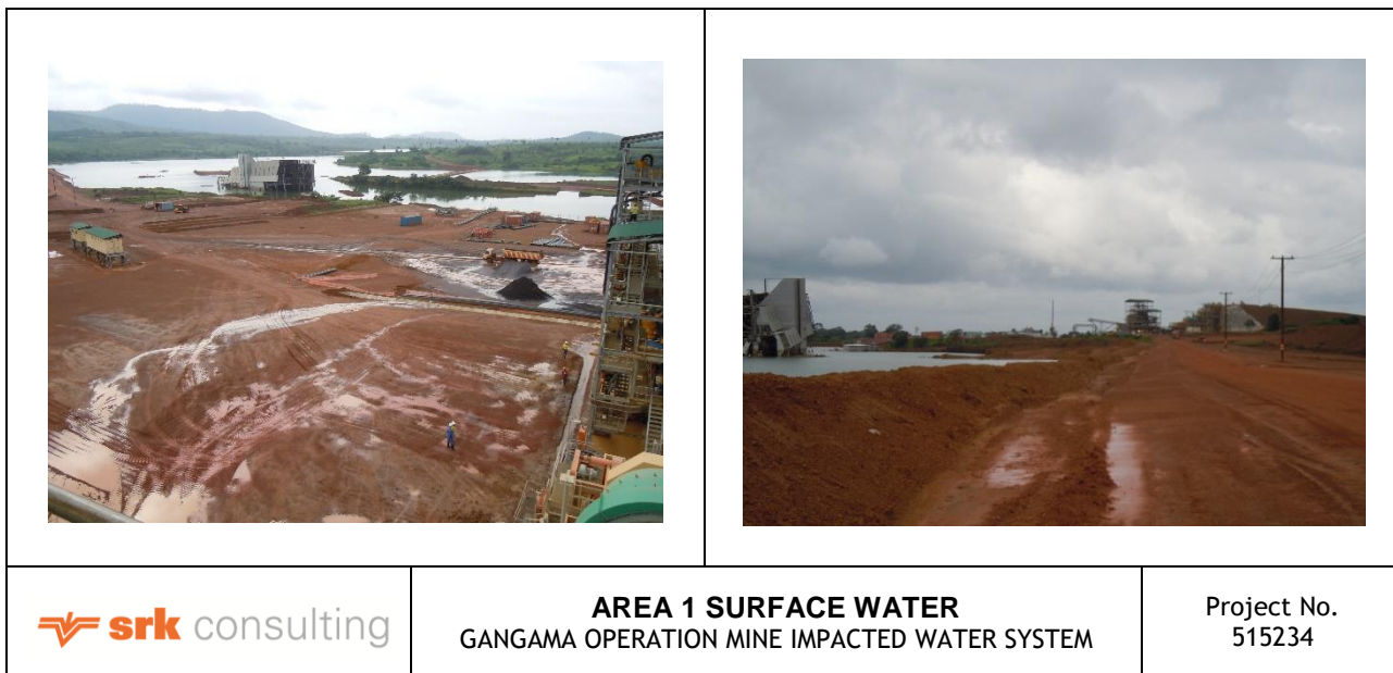
Figure 7-13: Photographs of the Gangama operation mine impacted water system
