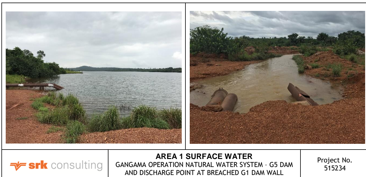
Figure 7-5: Photographs of the Gangama operation natural water system showing the G5 Dam (left) and the discharge point at the breached G1 Dam wall (right)
