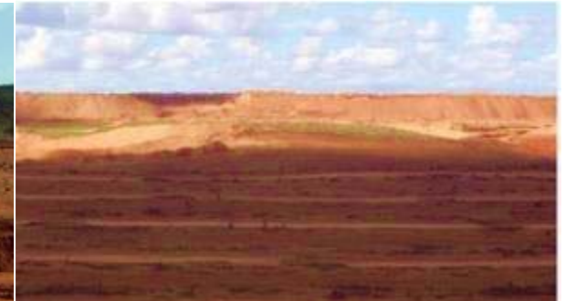
Cell 1 West 2014, rehab just completed
