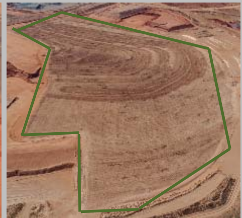
4. Southern tails storage facility
