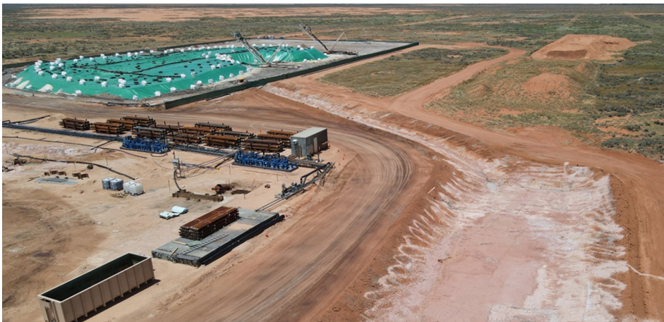
Figure 1 shows an aerial photograph of trial site.
