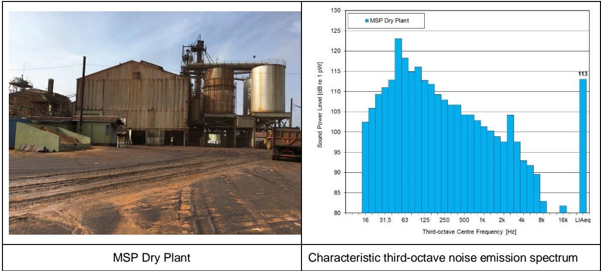
Figure 5-1 MSP Dry Plant noise emission characteristics
