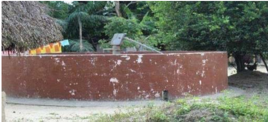
Figure 5.10 Hand pump water well in Foinda constructed by SRL
