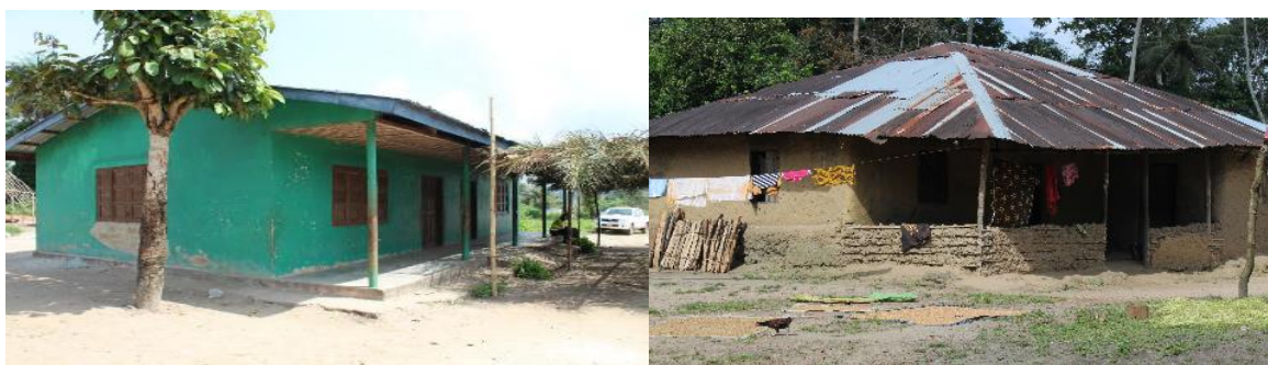
Fig 7.1 Typical structures to be replaced (Foinda Primary School left; typical house right)
