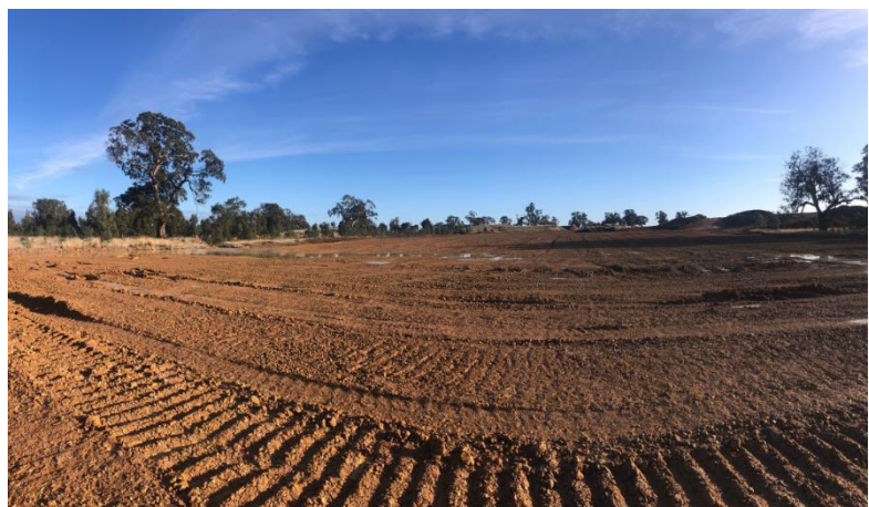
Pit 21 backfilled to design surface, April 2022
