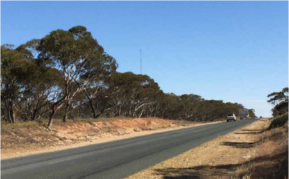
Photograph 25.2 Telecommunications tower adjacent to Balranald-Ivanhoe Road (photograph taken about 1 km from tower)
