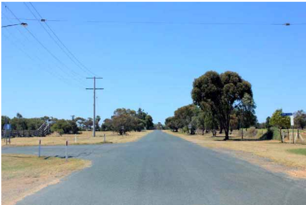
Photograph 3.15 Moa Street - O'Connor Street intersection (looking north from Moa Street)
