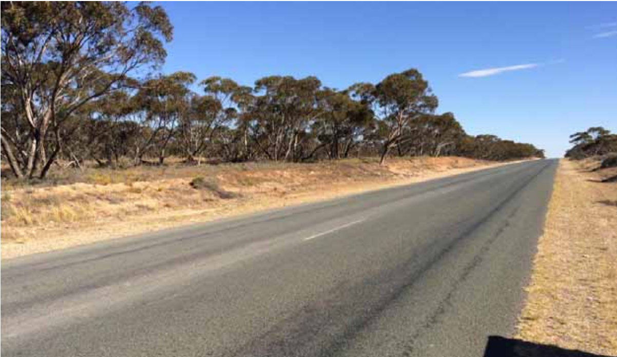
Photograph 4.2 Visibility at West Balranald access road intersection location looking south along the Balranald-Ivanhoe Road
