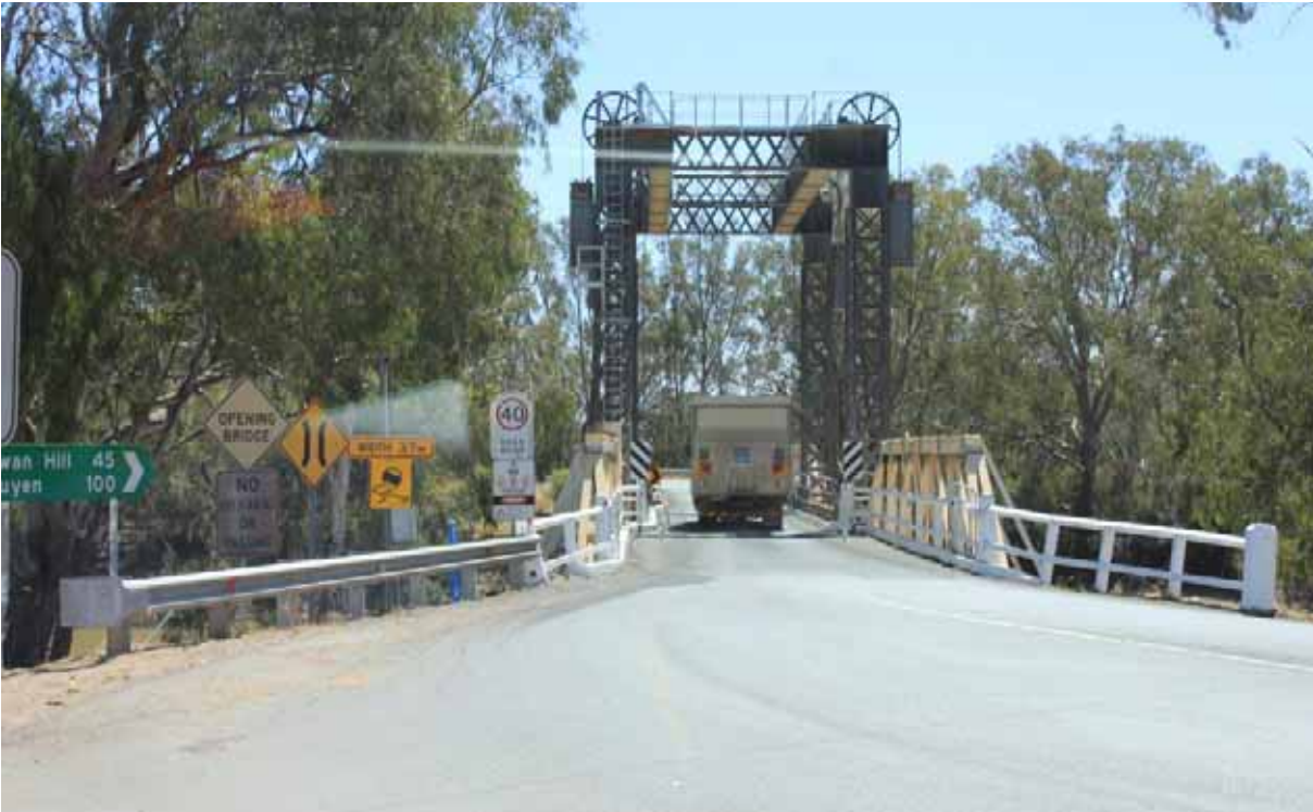
Photograph 3.12 Murray Street and Tooleybuc Bridge intersection (looking west towards the existing bridge from Murray Street)
