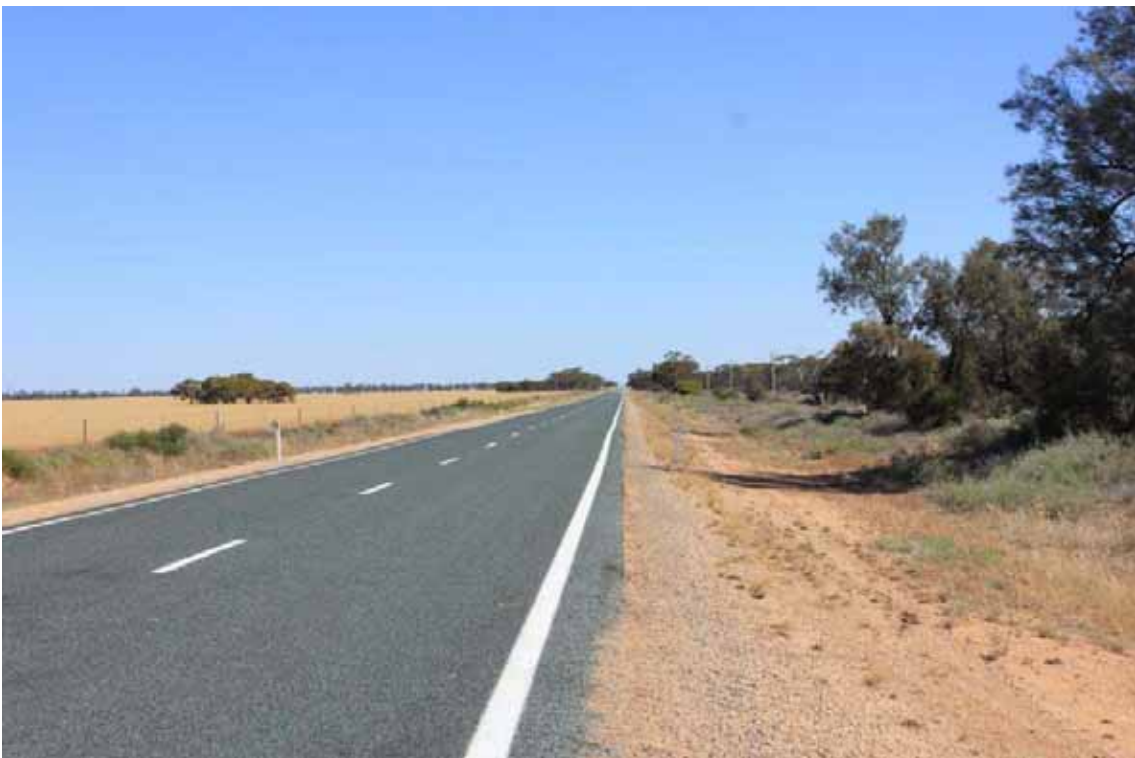
Balranald Tooleybuc Road Road 45 km north of Tooleybuc looking south
