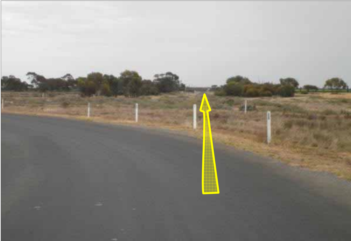
Photo A4 - Looking southwest along McCabe Street towards the McCabe Street / Sturt Highway intersection. Shows the wide pavement which exists outside K & SL Nelson Nominees Pty Ltd grain store operations, approximately 150m northeast of the Sturt Highway intersection. The traffic paths along McCabe Street have a lateral shift through this section of McCabe Street. At night the lateral shift is not clear and the correct through path not apparent for drivers.
