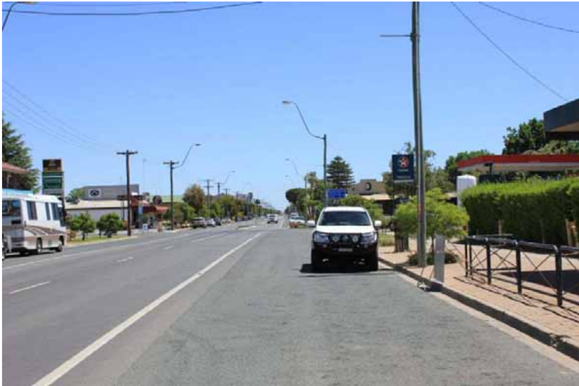
Sturt Highway (Market Street) at Balranald looking west
