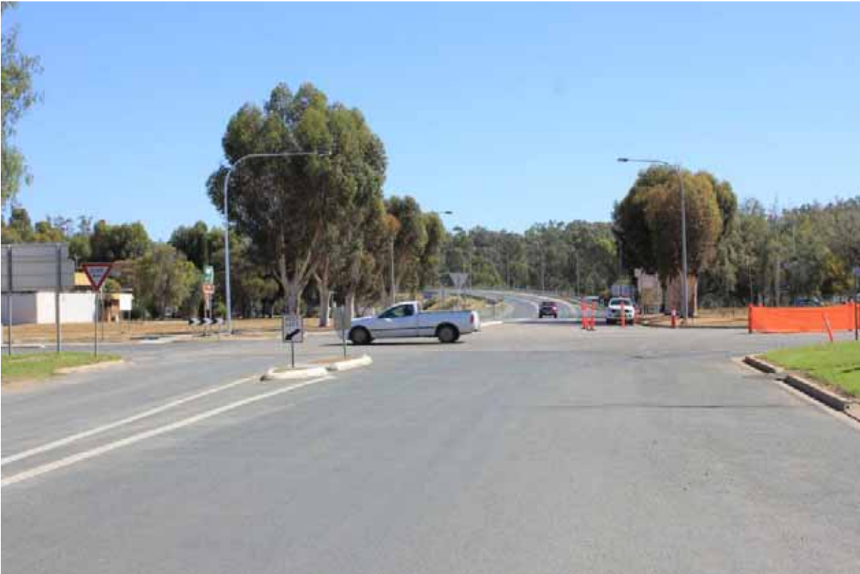
Photograph 3.6 McCabe Street at Sturt Highway intersection (looking south from McCabe Street)
