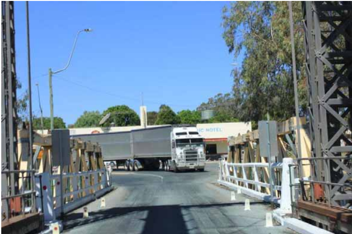
At Tooleybuc Bridge looking east
