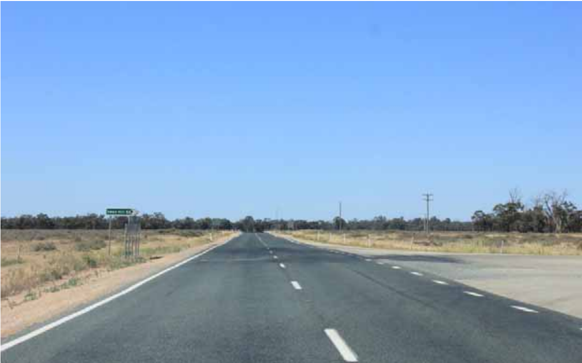
Photograph 3.10 Balranald-Tooleybuc Road - Swan Hill Road intersection (looking north from Balranald-Tooleybuc Road)
