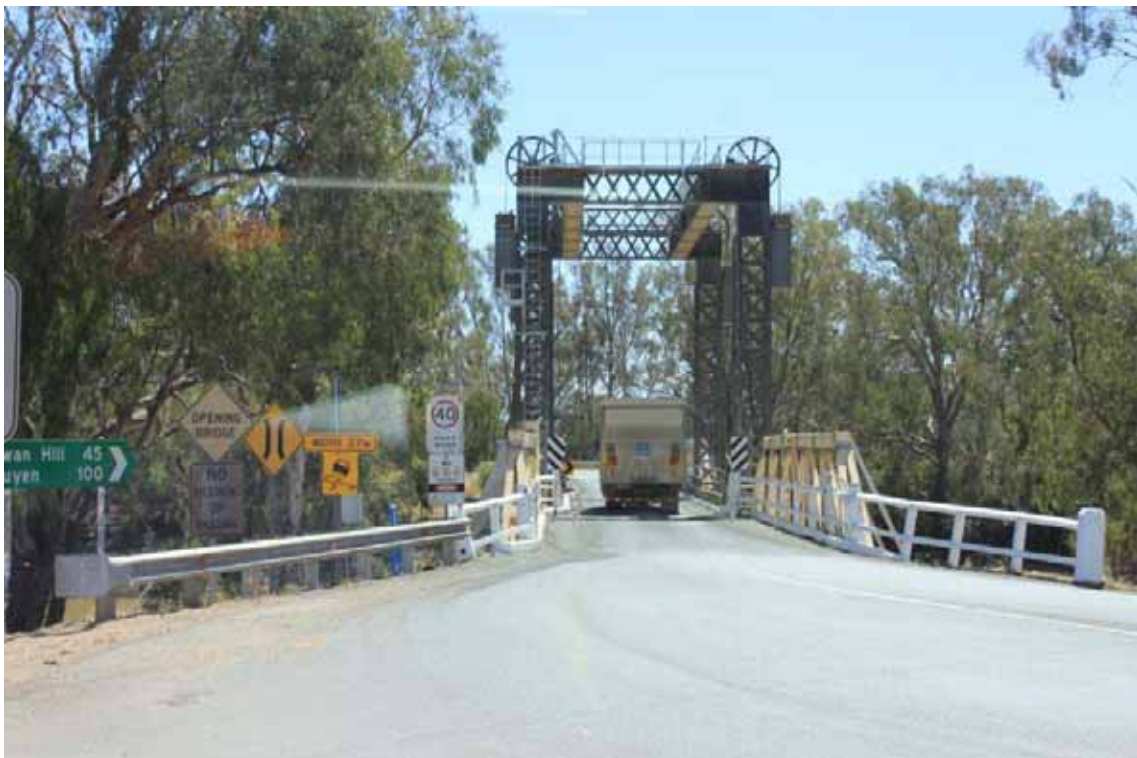
At Tooleybuc bridge looking west
