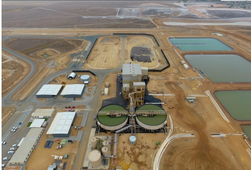
Large chloride ilmenite rich mine, commissioned in 2019. Ilmenite feeds synthetic rutile kiln with material zircon and rutile production.
