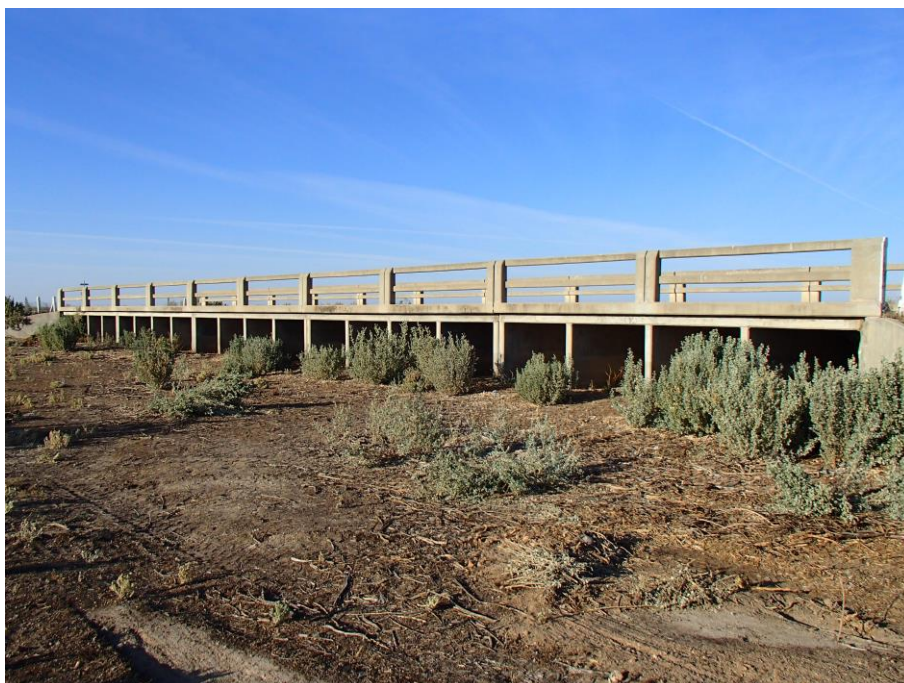
Figure 2.5 - Photograph of Box Creek culverts at Balranald Ivanhoe Road
