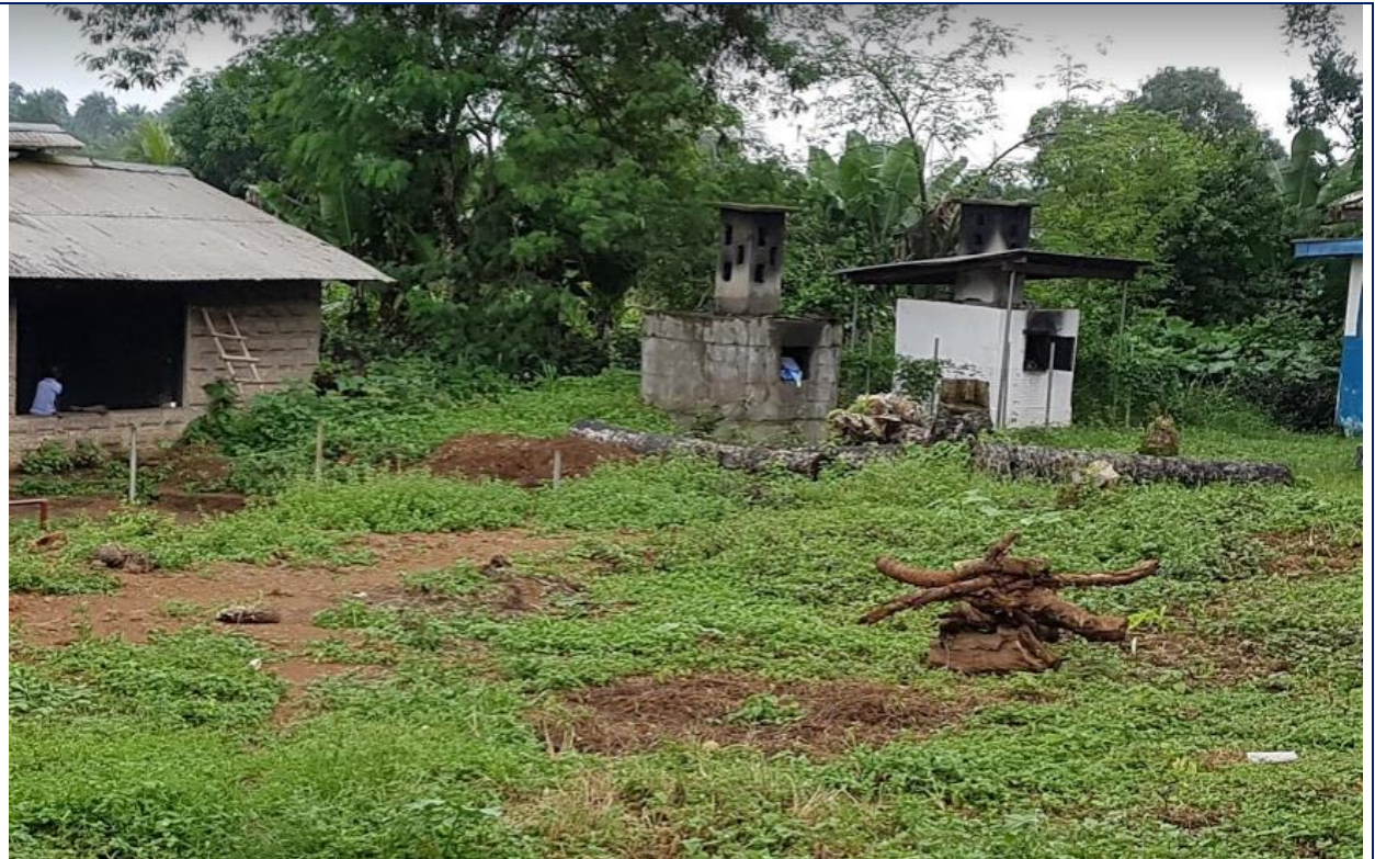
Incinerator at Mattru UBC
