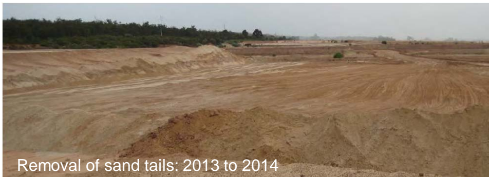
Replacement material: combination of clay fines, overburden and subsoil
